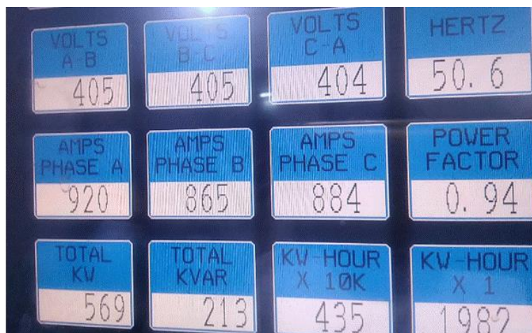
Figure 14: Operating frequency of gas engines
