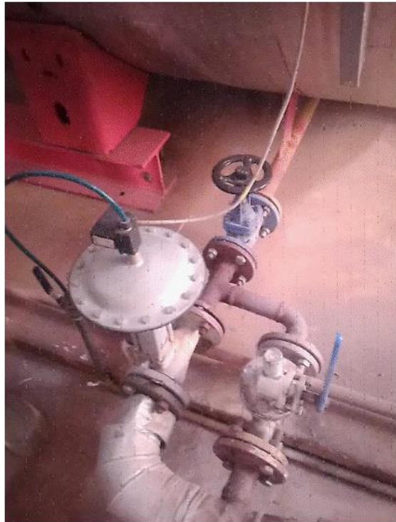
Figure 15: Manual blowdown practice
