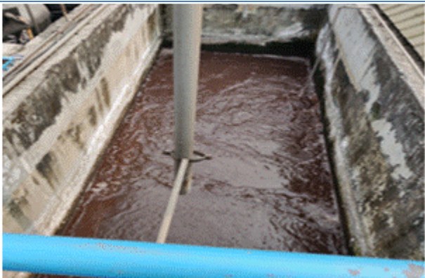
Sludge holding tank
