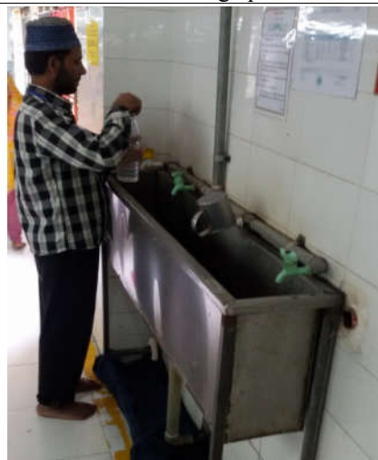
Installing push tap replacing ordinary tap
