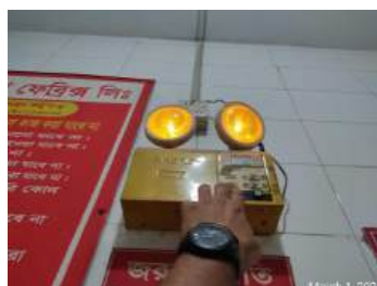
Testing emergency light.jpg
