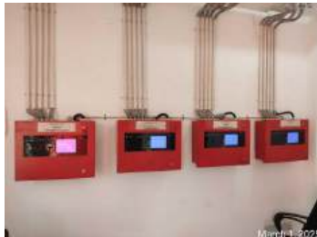
Fire alarm control panel.jpg
